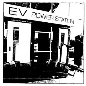
Nissan's Super-Quick Charger makes recharaing electric cars almost as easy as filling a gas tank. Motorists insert a computerized card, plug in the cord, and receive a 40% charge in six minutes or 100% charge in 15 minutes. The card provides vehicle charging requirements as well as billing information
