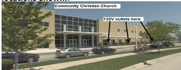
Community Christian Church in Naperville. At this upcoming meeting, for those who want to charge their PEV, drive up onto the sidewalk (YES onto the sidewalk!) and plug into one of the 120 VAC outlets <approximate locations shown.>
