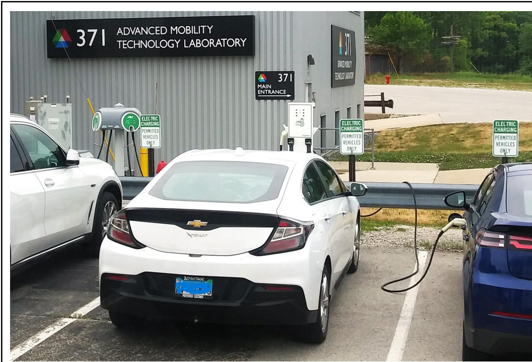
Onward to Building 371 with EVSE outside and EV testing systems inside
