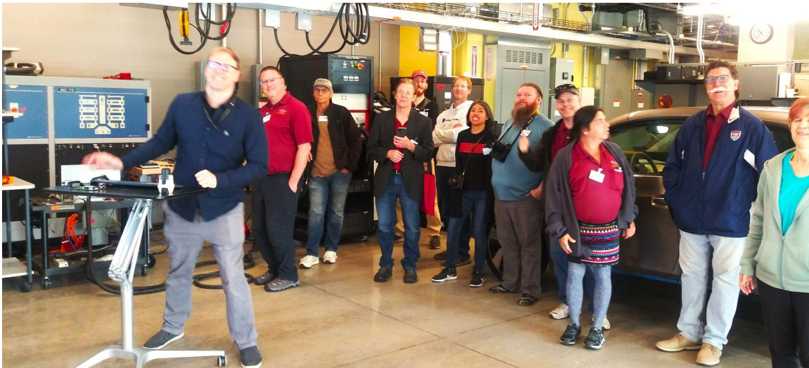
Mike shows us how, in a former gas station on site that was converted into an Electric Vehicle charging complex, how battery storage, canopies with solar panels, charging stations and external energy sources all interconnect.
