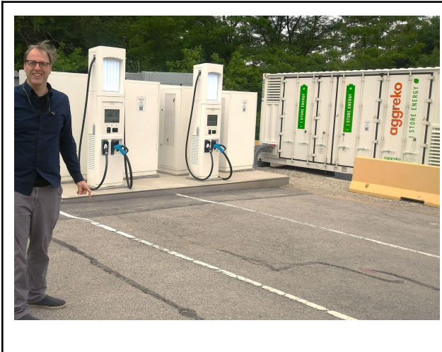
(Left) 350kW charging stations, and large scale battery energy storage system (BESS). Above Mike explains how the solar canopies, charging, power sources all connect and inter-work.
