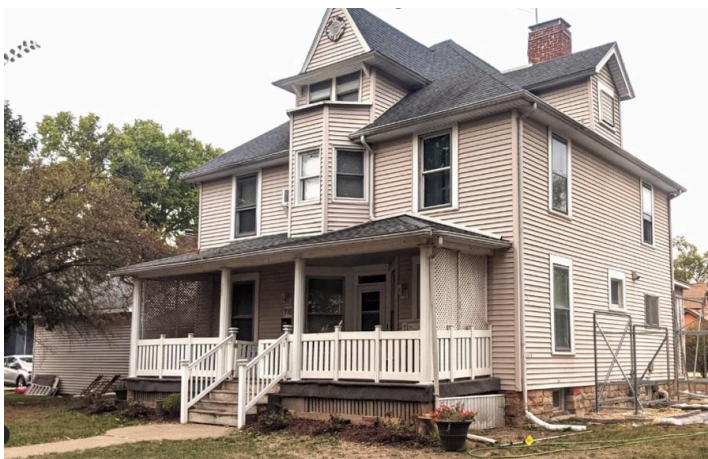
Jeff Miller's house - during renovation work in 2025
