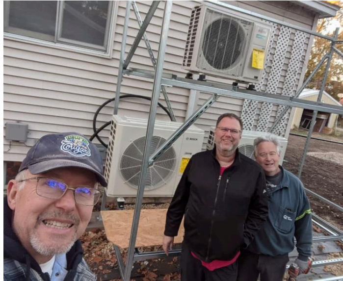
Installing the outdoor units. Bruce, Jeff, Rob
