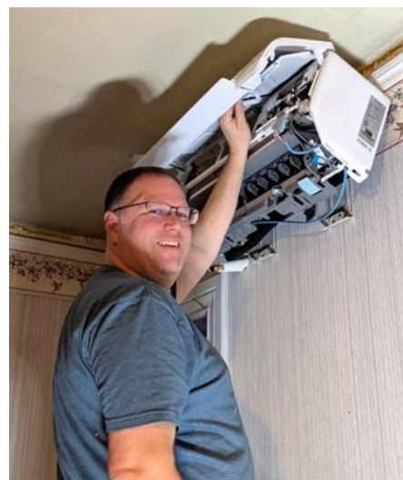
Jeff installing indoor heat pump unit
